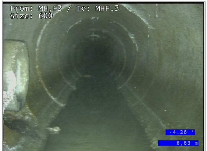
Connection at 9 o'clock, diameter 150mm
