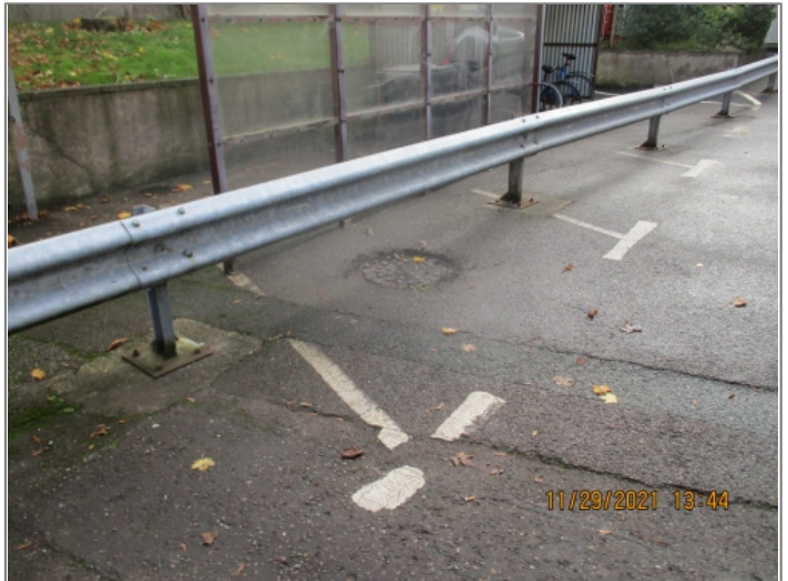
Manhole / Access Point: MHF,3 Location
