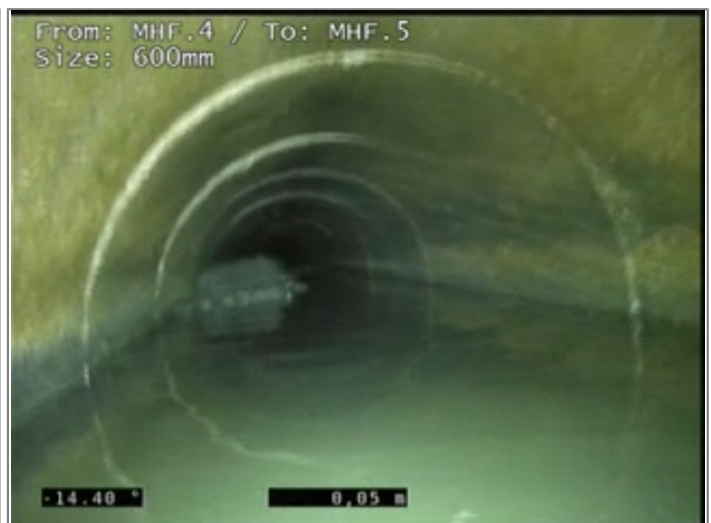
Survey abandoned - Remark: Camera unable to travel
