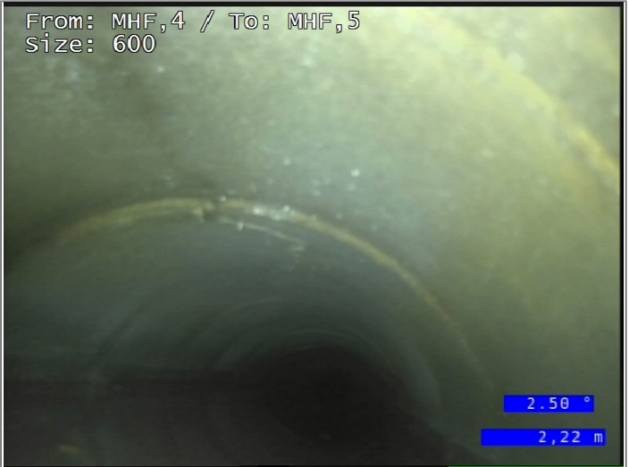
Debris Silt 50% cross sectional area loss
