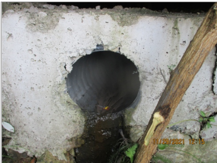
Manhole / Access Point: RIVER Internal
