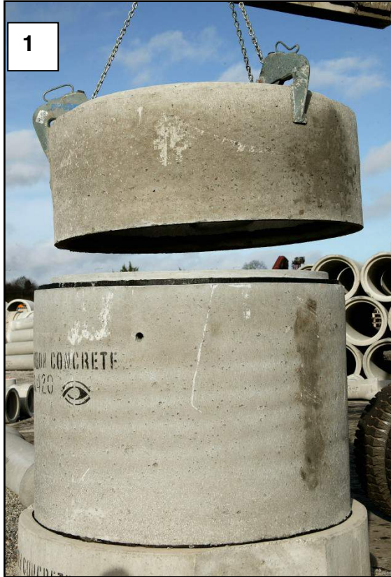
Positioning of 0.5M Chamber Ring
