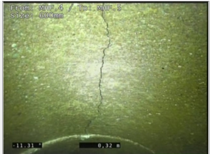
Crack longitudinal at 12 o'clock
