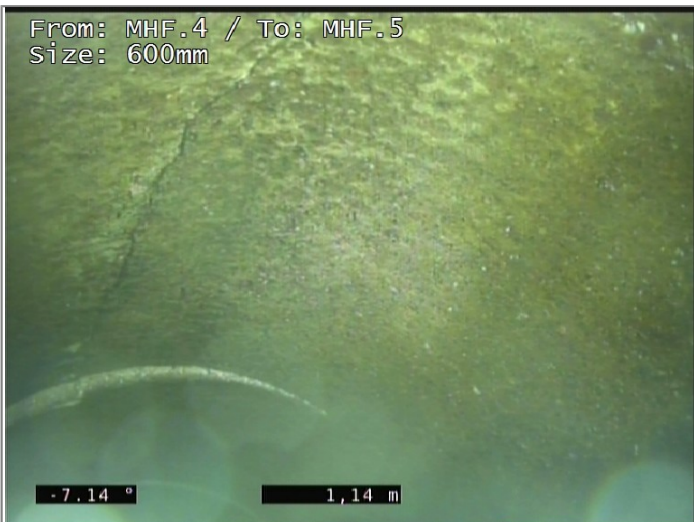
Survey abandoned - Remark: CAMERA WILL NOT TRAVEL...SILT DEBRIS IN DRAIN.
