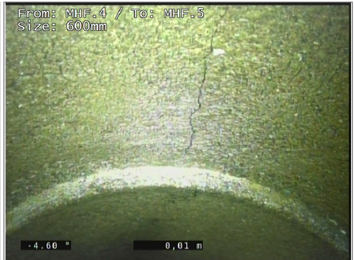
Crack longitudinal at 12 o'clock
