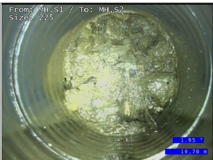
LINE LOOKS TO BE BLOCKED OFF
