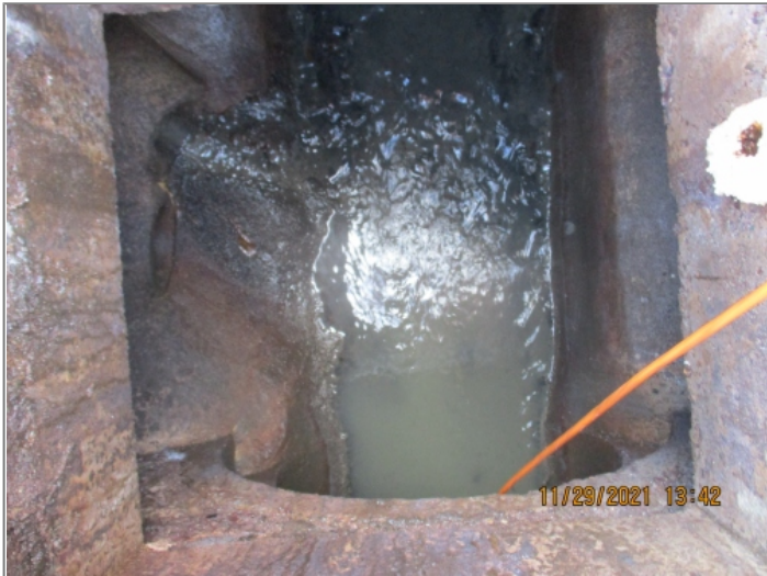
Manhole / Access Point: MH,F2 Internal
