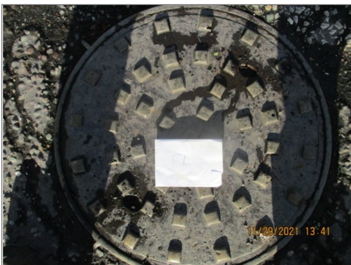
Manhole / Access Point: MHF,1 Internal - Unable to open
