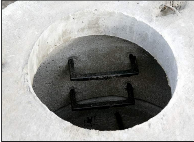
Manhole Cover Slab Showing Access Ope
