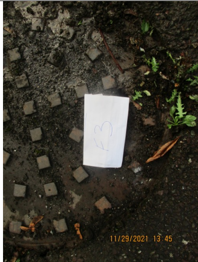
MHF,3 Internal - Unable to open, surface lifting with frame
