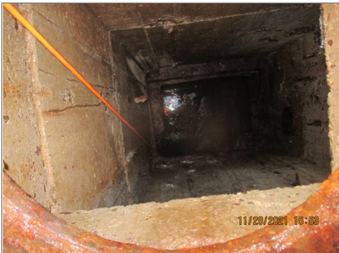
Manhole / Access Point: MHF,4 Internal
