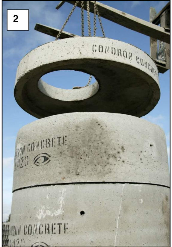
Positioning of Manhole Cover
