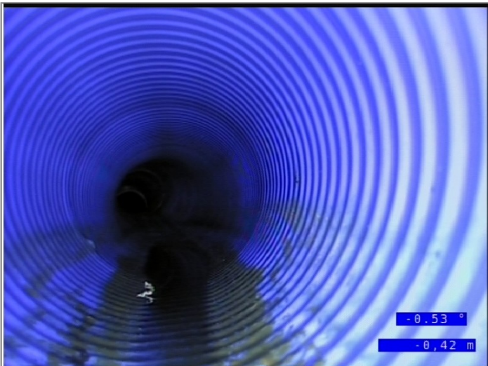
Start node type, manhole, reference MH.S1
