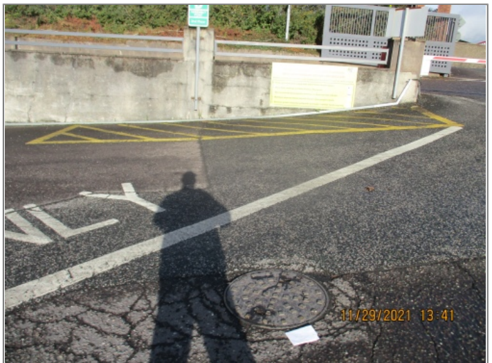
Manhole / Access Point: MHF,1 Location
