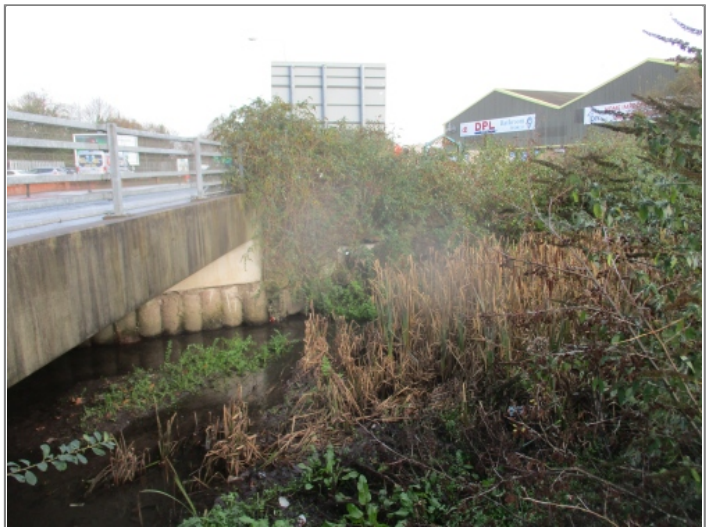
Manhole / Access Point: RIVER Location
