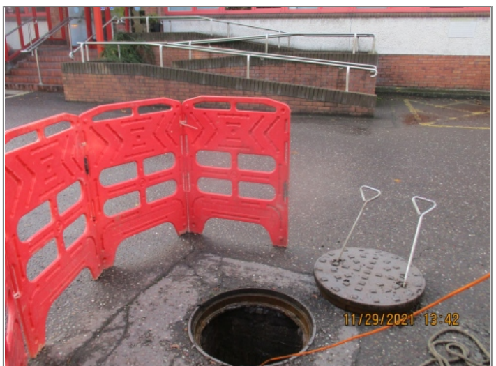
Manhole / Access Point: MH,F2 Location
