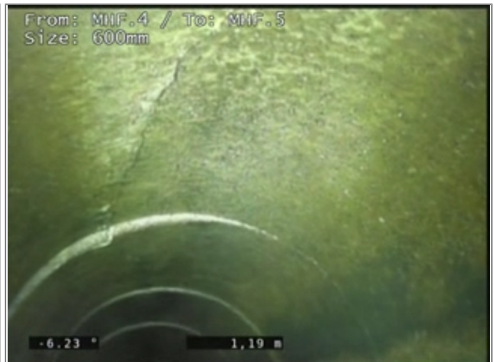
Crack longitudinal at 11 o'clock at joint
