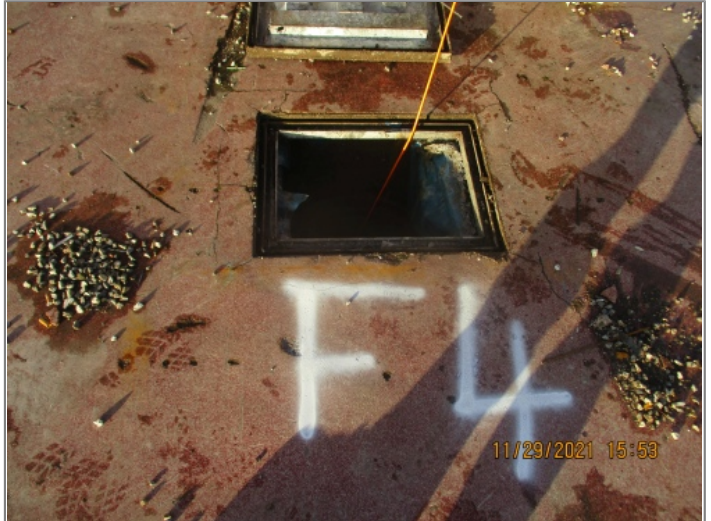
Manhole / Access Point: MHF,4 Location
