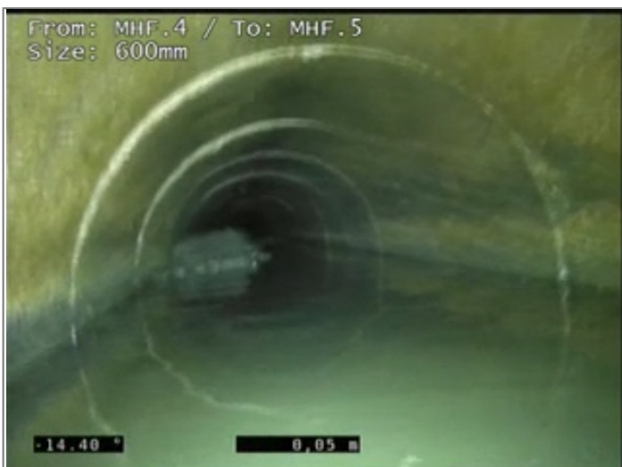
General observation at this point - Remark: Obstruction in pipe 3 meters D/S Possible concrete block
