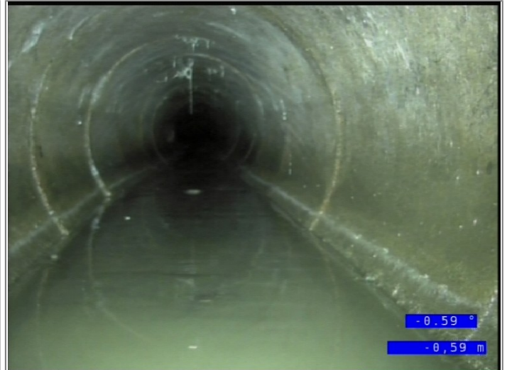
Start node type, manhole, reference MH,F2
